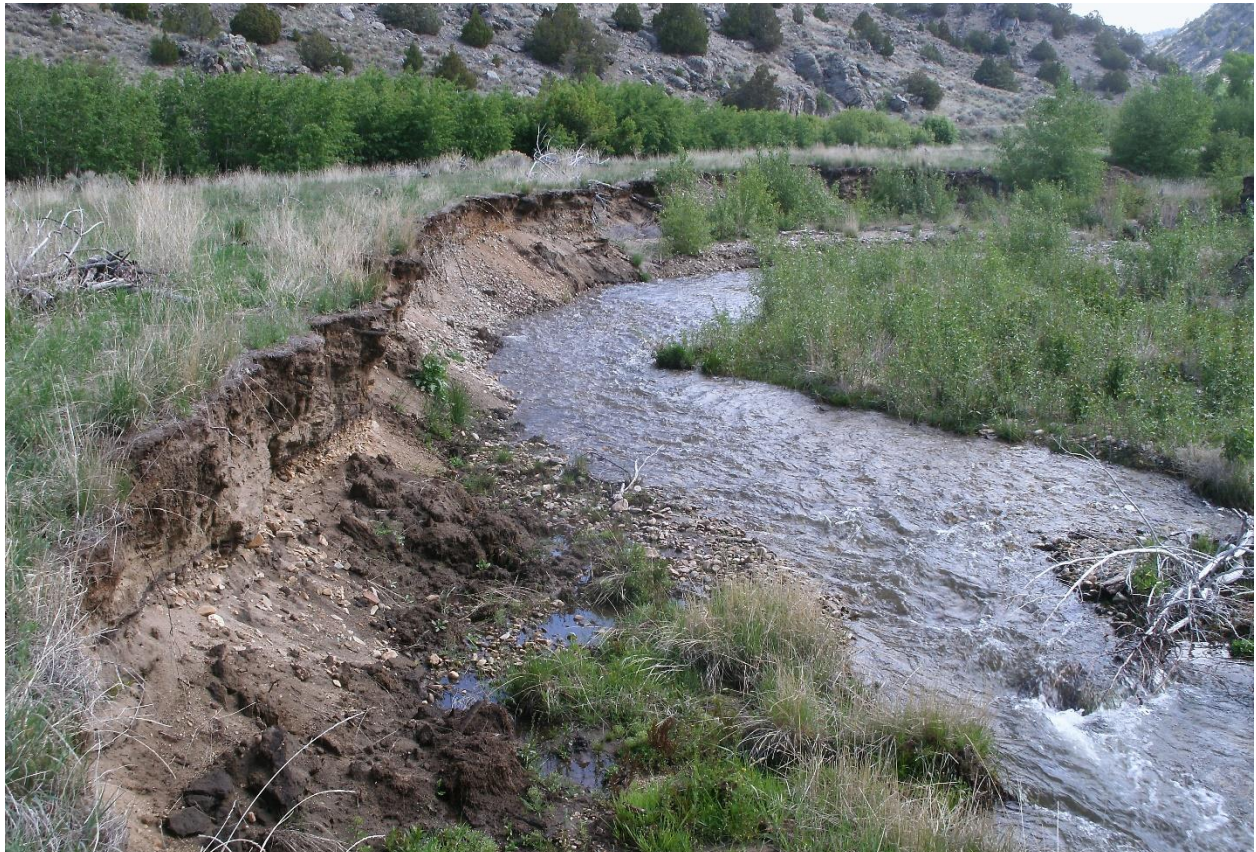
Figure 8: Example of historical mining resulting in restricted floodplain and erosive banks on Ramshorn Creek. Placer deposits can be seen perched above the stream channel on the left
