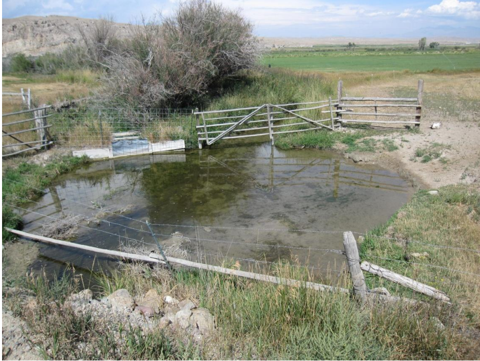
Figure 3. Lower Spring Creek. Start of the lower 0.5-mile reach just below East Bench Road. Cattle access has over-widened the channel, causing sediment deposition. The irrigation control structure is blocking the stream from fish passage. (Photo, August 2013)
