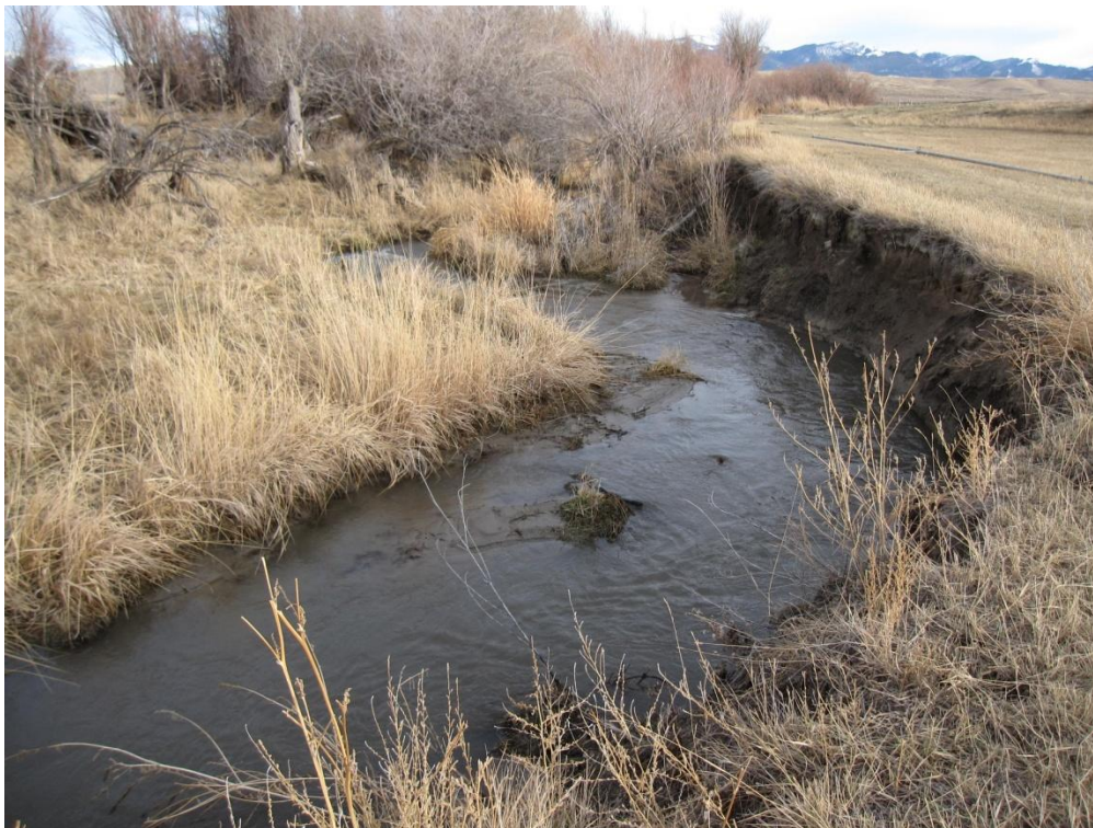
Figure 4. Lower Spring Creek. Channel banks are eroding from lack of vegetation. Riparian fencing is needed to prevent cattle access to the stream. (Photo, November 2012)
