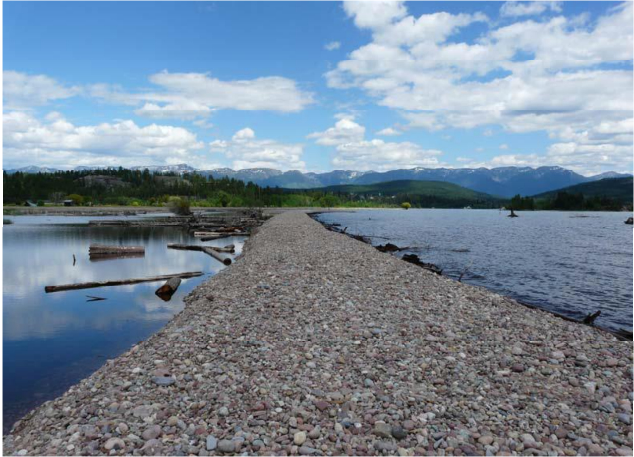
Example of completed offshore dynamic gravel beach with spit at end of structure.
