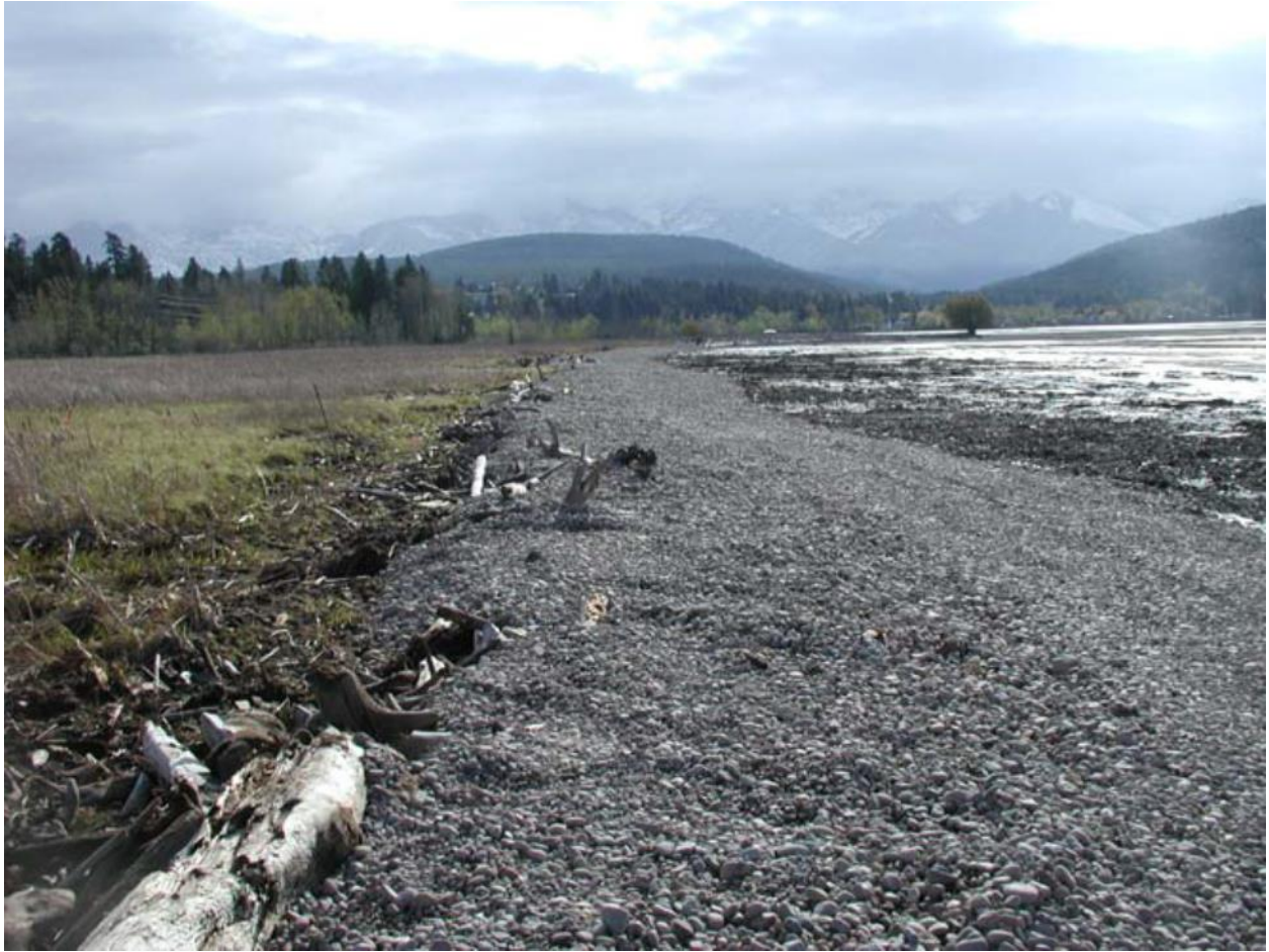
Example of finished shore attached dynamic gravel beach before wave action during full pool lake levels.
