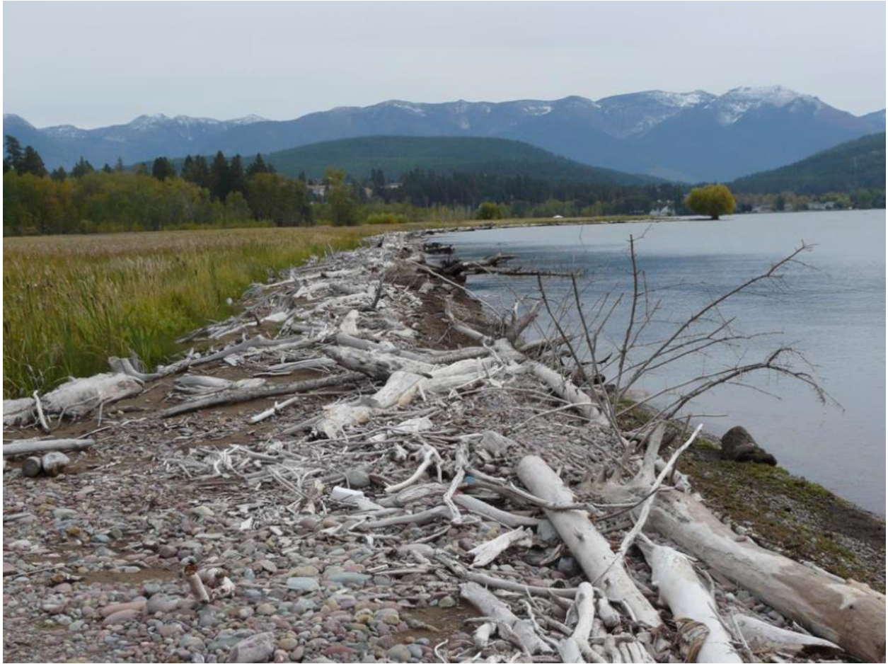
Example of attached dynamic gravel beach after 3 full pool seasons of wave action. Note: All wood on the beach was delivered to the beach by waves and that overtopping during storms occurs maintaining the process of connectivity with the wetland.
