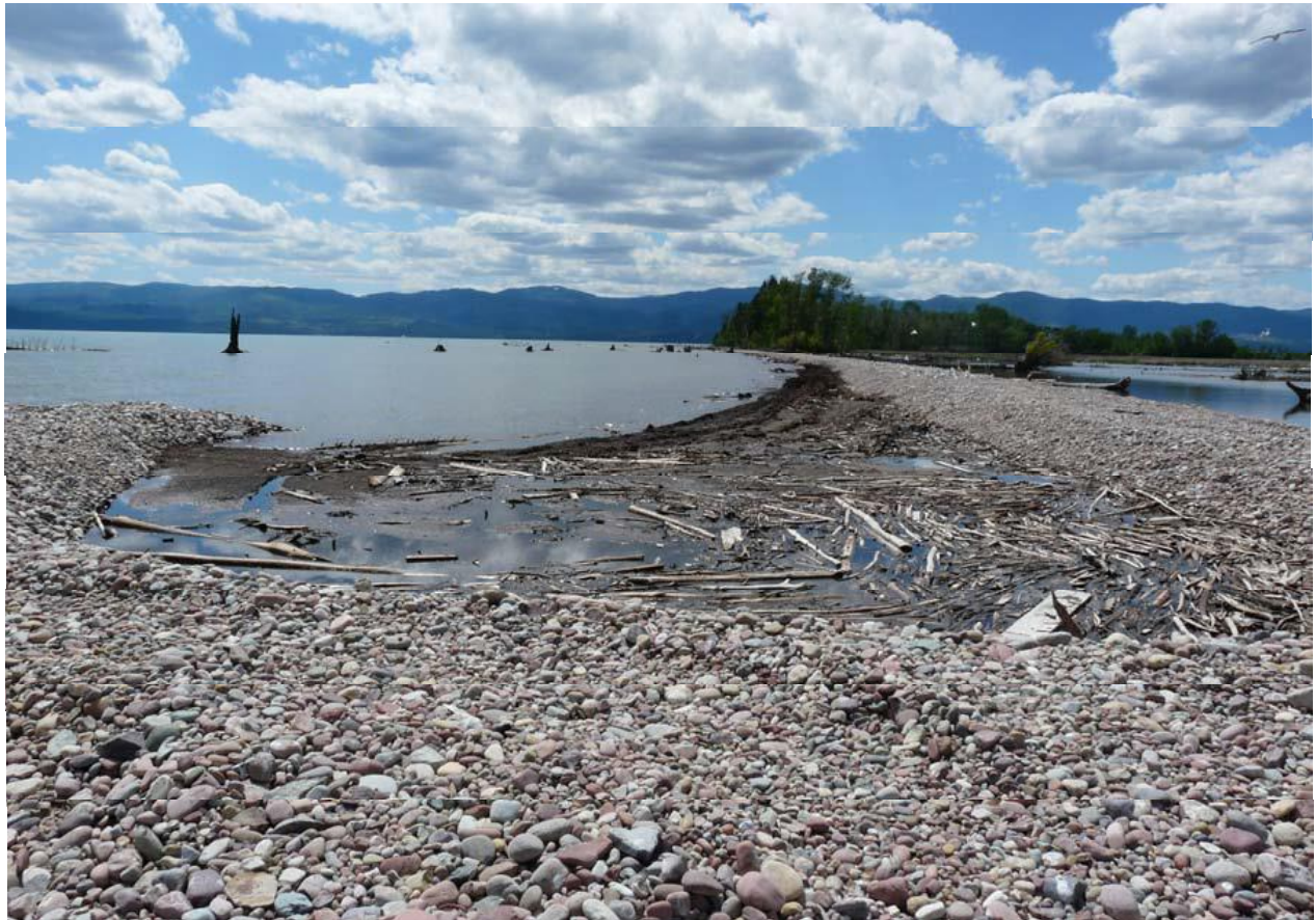
Example of offshore dynamic gravel beach spit embayment after construction and a few weeks of full pool lake levels.
